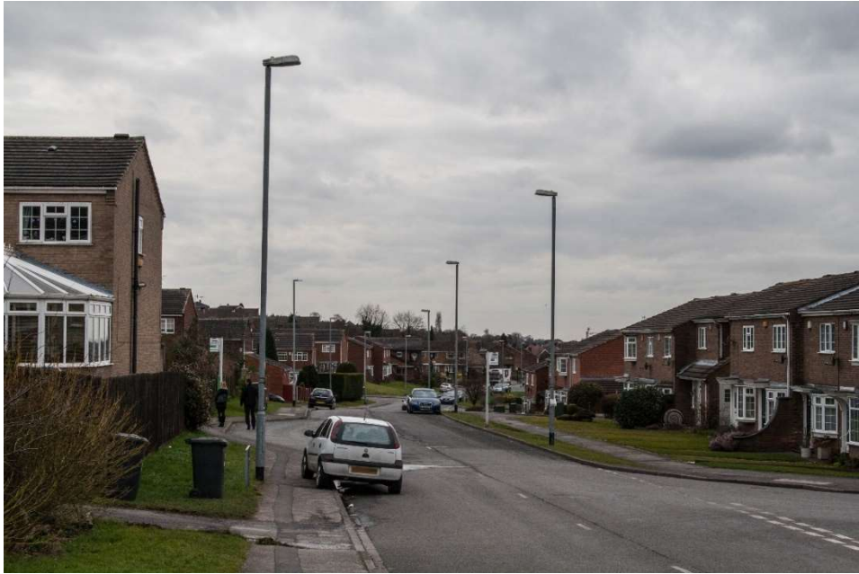
Terraced 1970's residential development on Howbeck Road with limited enclosure and a generally homogenous character
